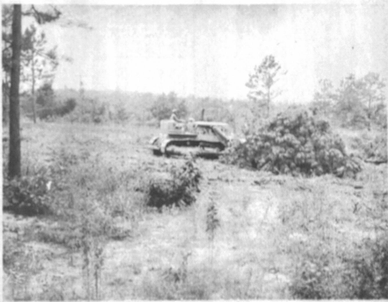
IT'S STARTED—Construction on the new Tishomingo county courthouse got underway this week with preparation of the
